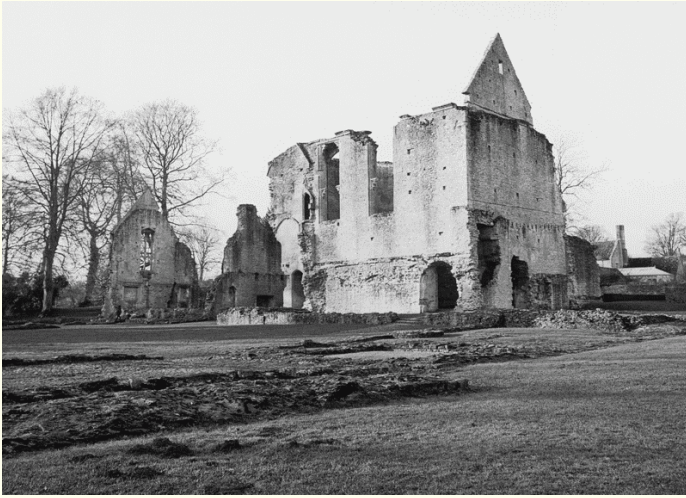
Minster Lovell Hall from the south-east in 2000, showing surviving hall range.
