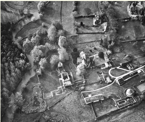
Minster Lovell Hall and church looking west, showing former vicarage house (top center), Hall, church, and Manor Farm (center), and Manor Farm's farmyard (bottom right)
